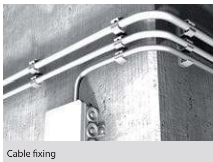
Fixing plastic insulating conduits
